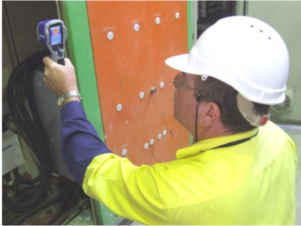
A thermal imaging inspection being carried out.
